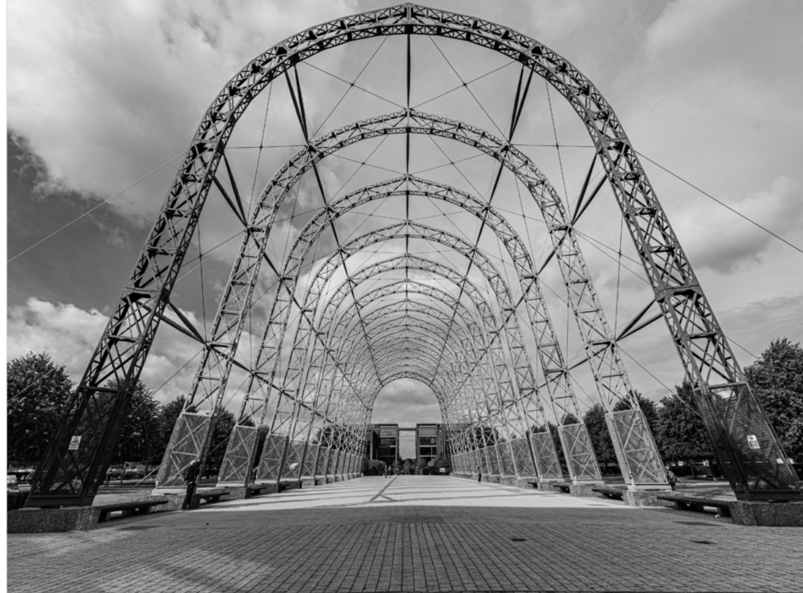
"Airship Hanger, Farnborough Airport" Graham Chisnall
